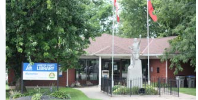
New exterior signage with Lambton County Library and municipal partner branding installed at the Alvinston Library.
